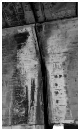
**Figure 6.** Joint of span and approach structure
