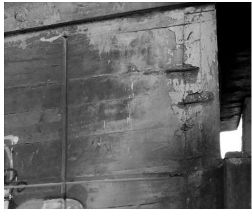
**Figure 7.** Visible reinforcement – wing wall III
