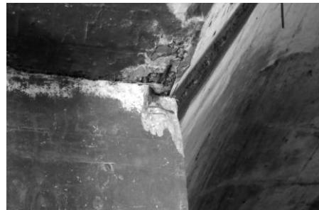
**Figure 9.** Crushed concrete on bearing-abutment in axis A
