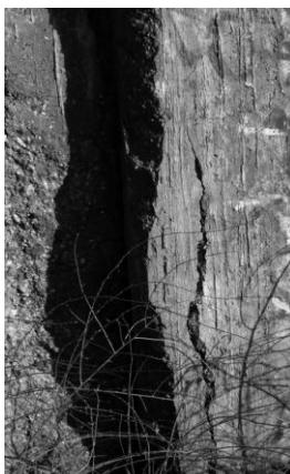
**Figure 8.** Vertical crack and mechanical damage-abutment in axis D
