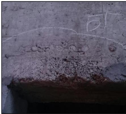
**Figure 9.-Concrete segregation and breaking of corners**
