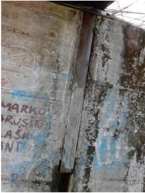
*Figure 13. Damaged drainage installation, leakage of water, biological corrosion*
