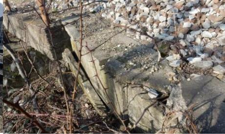
*Figure 17. Damages of precast pedestrian walkway slabs*
