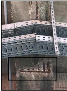
**Figure 16.-**Visibly scratched reinforcements
