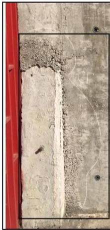
**Figure 14.-**Concrete segregation
