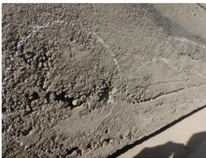
*Figure 8. Wall panel - Concrete segregation and visible reinforcement*
