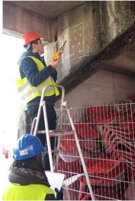
**Figure 20.-Schmidt hammer testing process**
