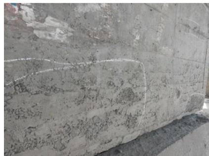
*Figure 9. Formwork traces, adhesion between concrete and framework*
