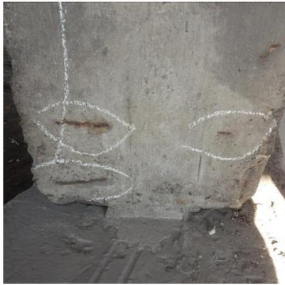
*Figure 6. RC wall - insufficient thickness of the protective layer visible corroded reinforcement*
