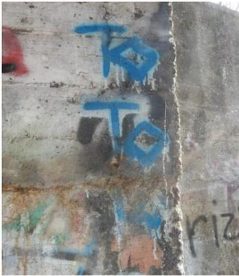
*Figure 5. RC wall - Uneven edges, rust leakage, improper horizontal break of concreting*
