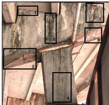
**Figure 12.-** 1)Cracks in the places where the precasted elements are suspended, 2) Corrosion of steel reinforcements, 3) Biological corrosion of concrete, 4)Color change due to water spillage, 5) The first form of chemical corrosion (flushing  $\text{CaCO}_2$ ), 6) Damage due freeze-thaw cycle
