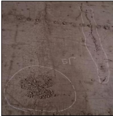
**Figure 8.-Concrete segregation**
