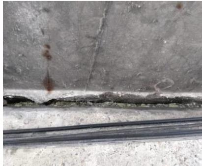
*Figure 12. Crack and crumbling of concrete at the joint of main girder and retaining wall, corrosion of reinforcement*
