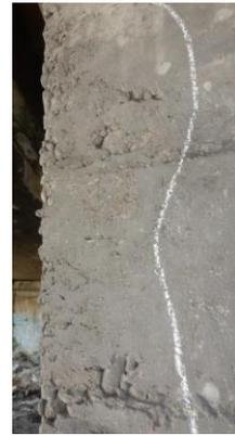
*Figure 7. Honeycombing on wall panel*
