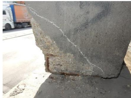
*Figure 15. Delamination of the concrete in the lower parts of RC wall, friable concrete, corrosion of reinforcement*
