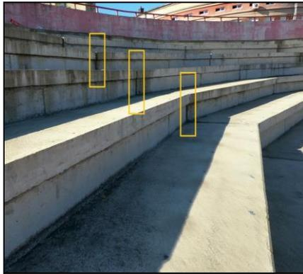
**Figure 18.-**The inadequate connection between the panel and the tribune
