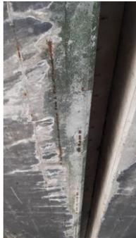
*Figure 11. Water penetration, stains on the surface, reinforcement corrosion on expansion joints between main girders, leaching of  $\text{Ca}(\text{OH})_2$*
